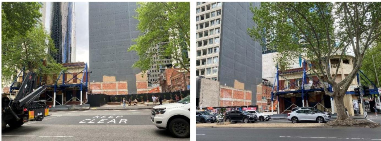
Figure 5: Demolition on site has commenced this permit (Source: Planning report by applicant)
