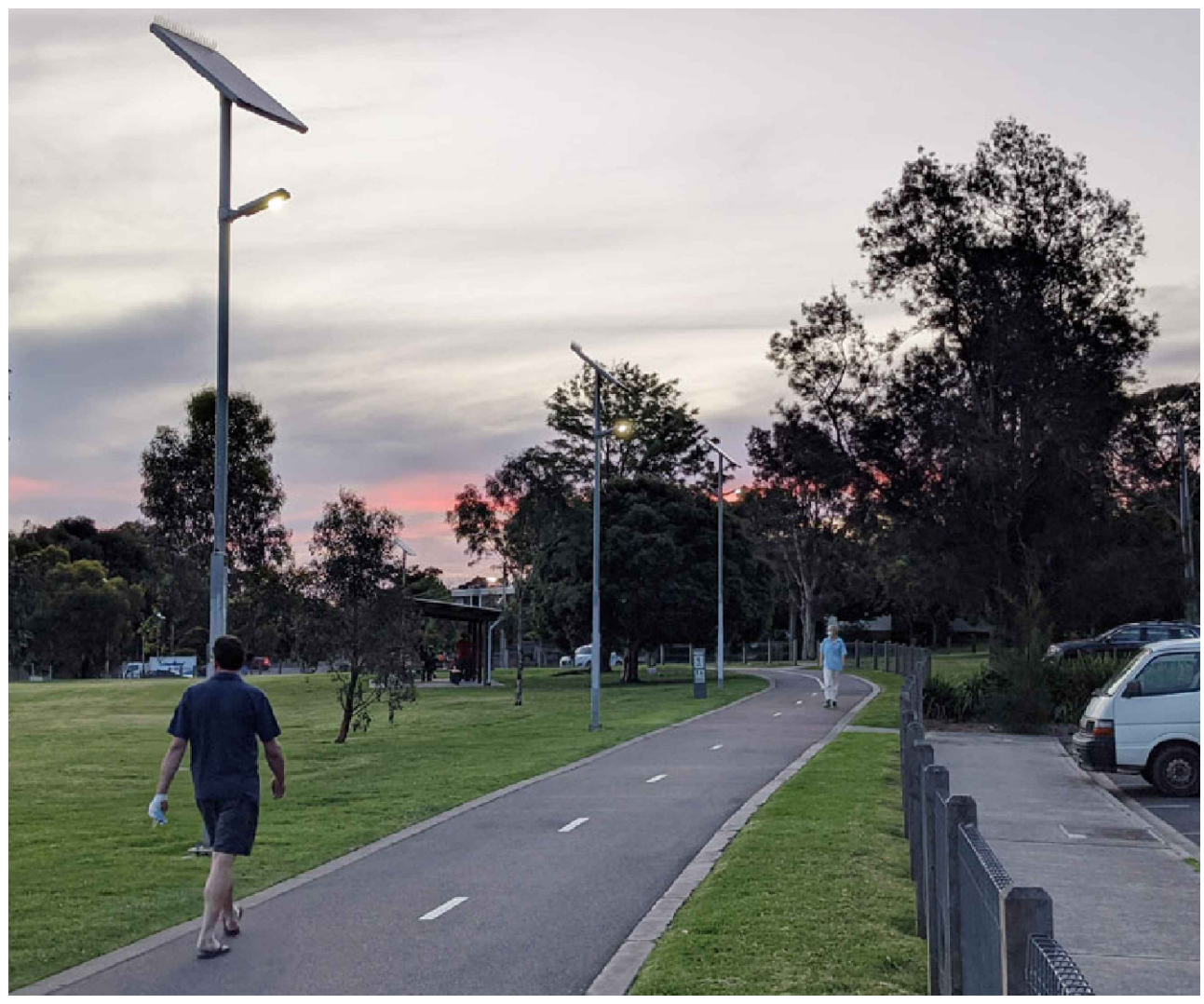
LIGHTING ARRANGEMENT LIGHT POLES TO BE LEADSUN OR APPROVED EQUIVALENT. ALL EXTERNAL LIGHTING CONTROLLED VIA PE-CELL AND TIME CLOCK.
