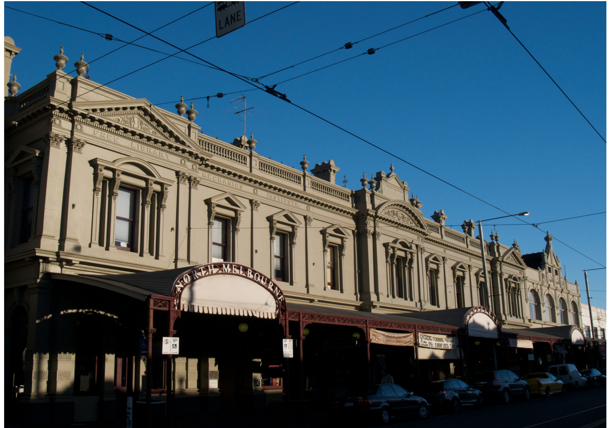
Figure 13: Historical Buildings on Errol Street, North Melbourne (Source: fredodonnellphotography)
