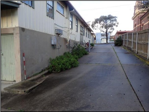
Plate 3: View of the driveway with slope, facing south (photo by J. Hardy, 5/12/2019)
