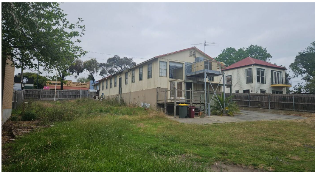
Figure 2: The extensive lawn area and rear of the existing building.
