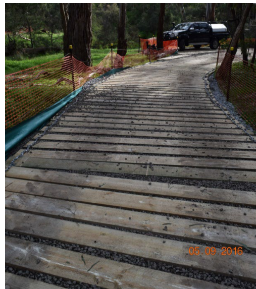
Figure 9: Rumble boards over crushed rock.
