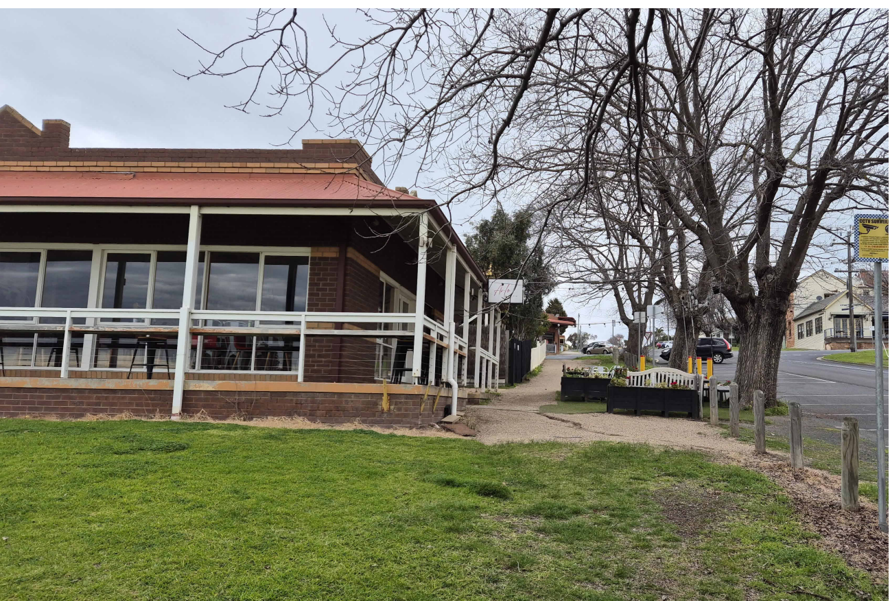
IMAGE 7 LOOKING SOUTH, 1 HARDING STREET
