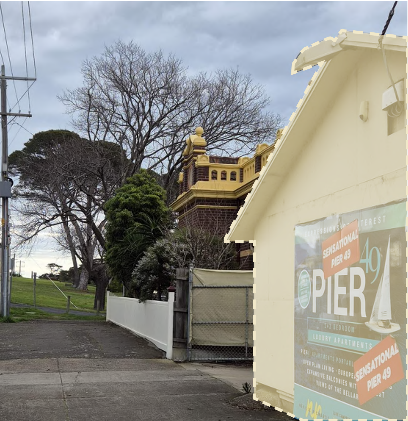
View of Existing Building
