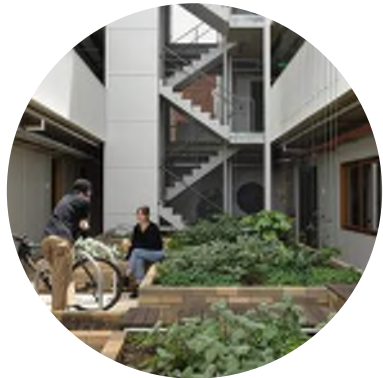
Breezeway circulation and dual-aspect apartment allows for cross-ventilation and reduced cooling loads
