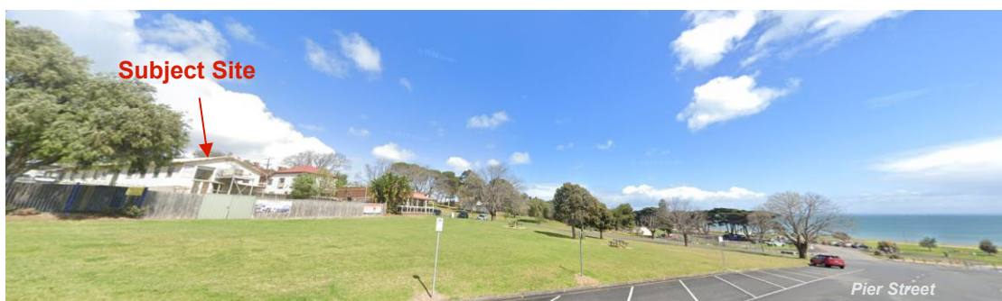
Figure 5: Streetscape view of Foreshore Reserve
