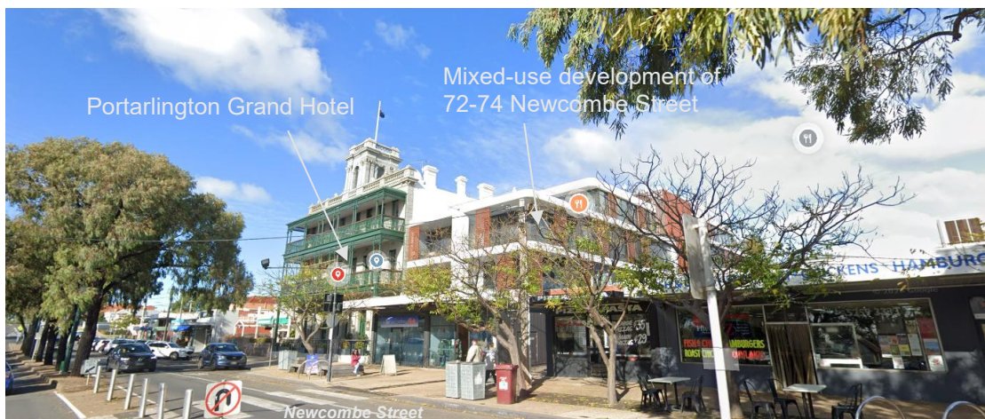
Figure 9: Streetscape view of the mixed-use development at 72-74 Newcombe Street
