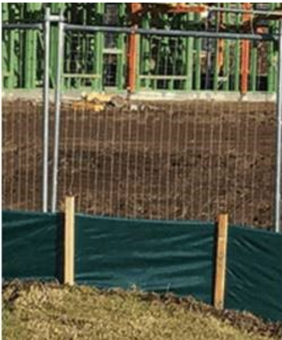
Photo 8 Example of temporary fence with silt fence (green material) for Swamp Skink mitigation.
