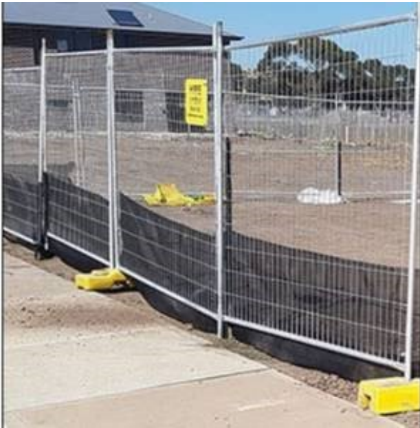
Photo 7 Example of temporary fencing and silt fence (black material) for Swamp Skink impact mitigation.
