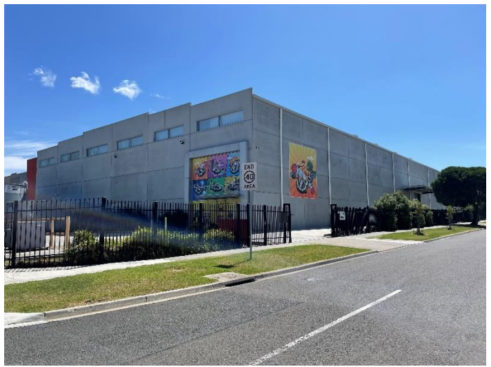
Figure 6: View of 50 McArthur Street – go karting premises
