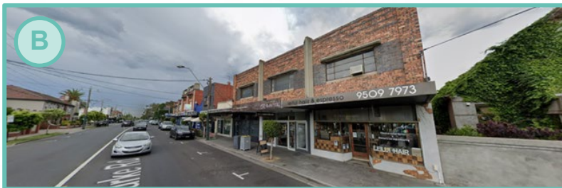
Picture 4 Burke Road Commercial Strip
