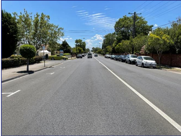
Figure 11: Burke Road – view north
