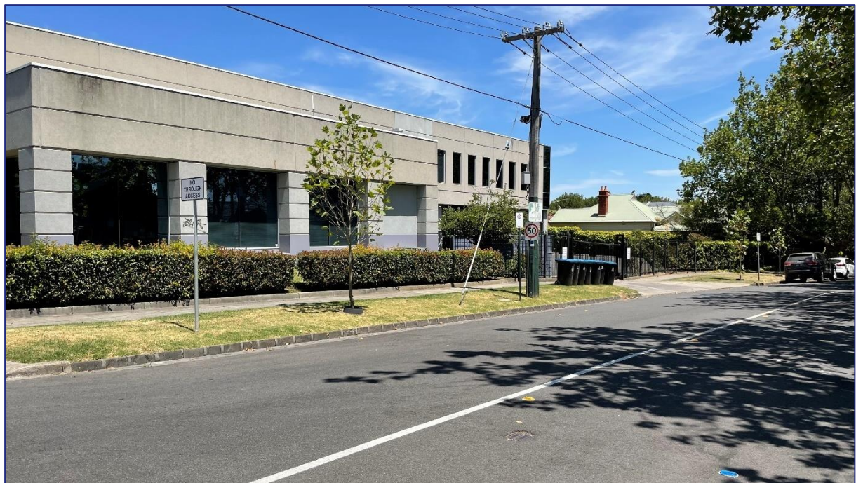
Figure 7: Subject site (view south-west from Hope Street)
