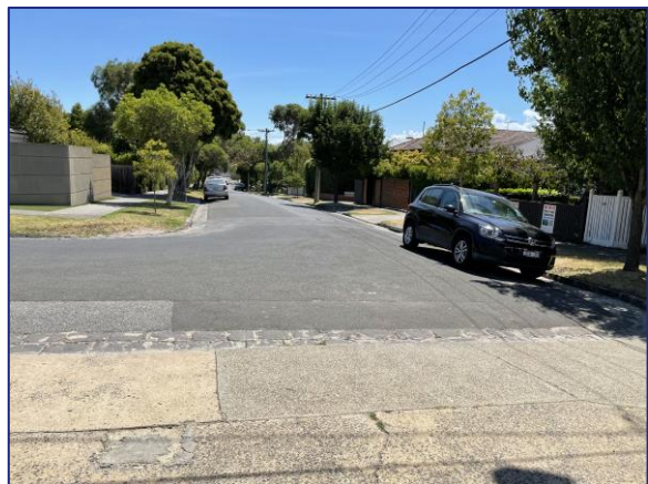
Figure 9: Irymple Avenue – view west in the vicinity of ROW
