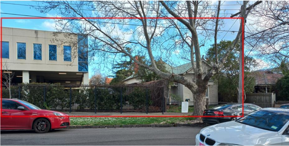
Figure 9 Subject site from Hope Street
