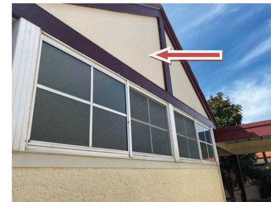
Toilet block gable infills – no asbestos detected
