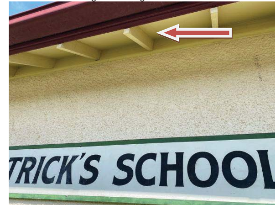
Rear of original building eaves – no asbestos detected
