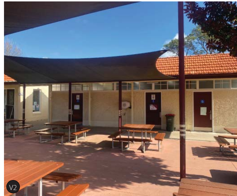
V2 Shaded seating area and toilet amenities block.
