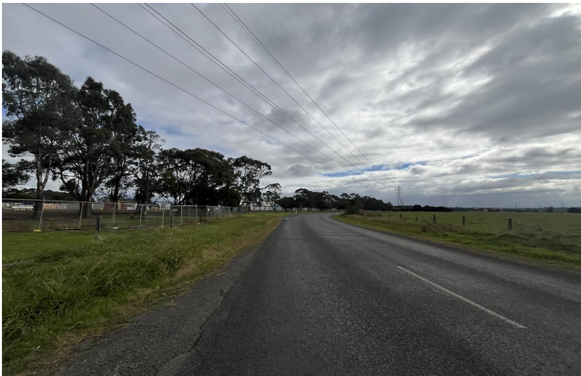
Figure 5: View along Bonds Lane, looking west toward the subject site on the right. The land on the southeastern side (left) comprises the proposed Wooreen Battery Energy Storage System (BESS), currently under construction.
