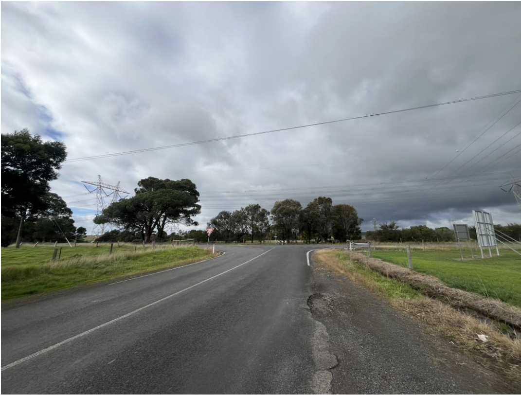
Figure 6 : View towards the Tramway Road and Bonds Lane intersection, showing the subject site to the left and the proposed Wooreen BESS site to the right.
