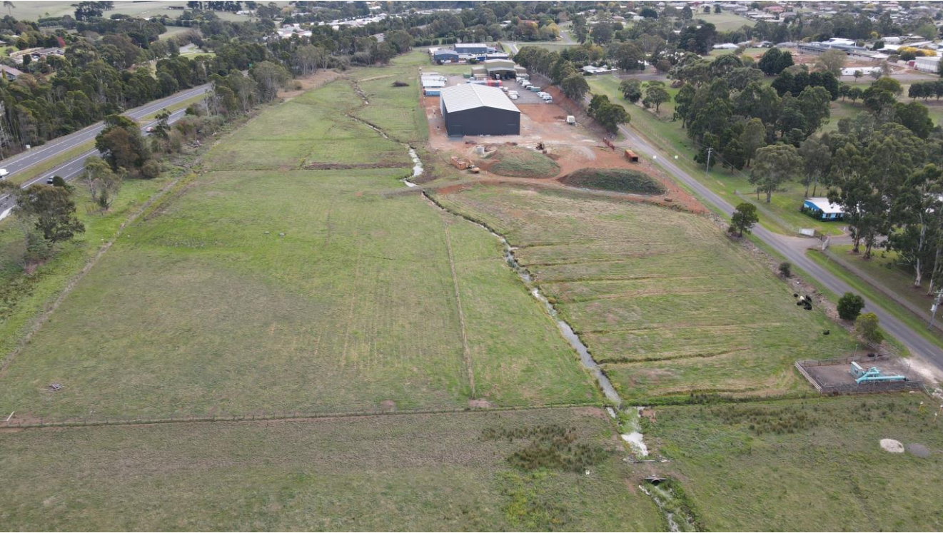
≈ Whole site from East
