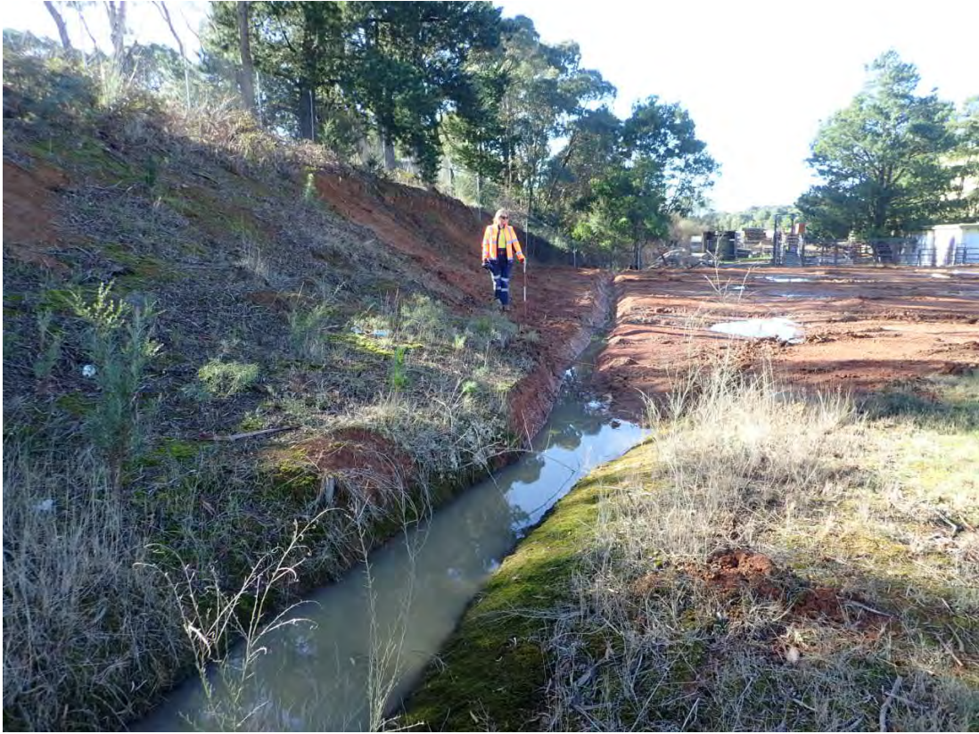
Plate 1. Batter up to 4 m high on south side of Wills Street. View to east.
