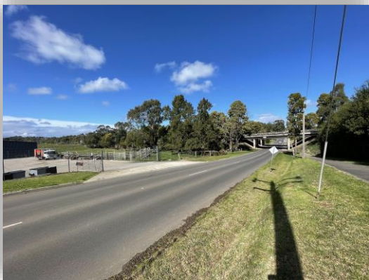
Figure 2.6: King Street, looking south
