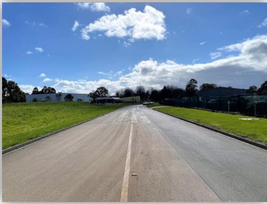
Figure 2.4: Spring Street, looking north
