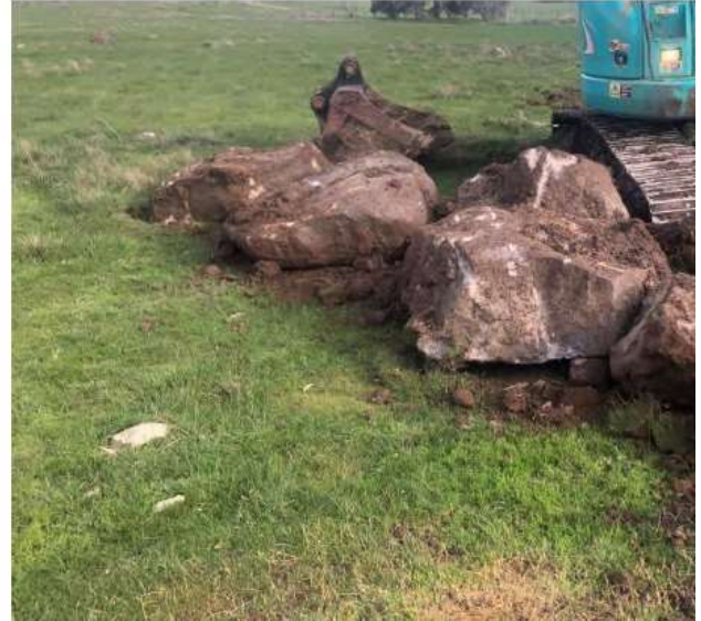
FIGURE C-2 TP 115 SHOWING SHALLOW ROCK
