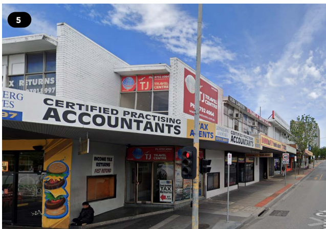
Figure 05: View of Clow Street streetscape looking west
