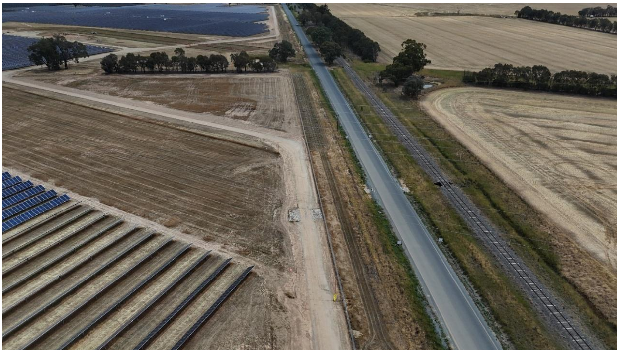
FIGURE 2-3 NORTHERLY AERIAL VIEW OF PROPOSED BESS AREA (ENGIE, 2025)
